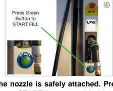
The nozzle is safely attached. Press green START button and hold until fill in completed.
